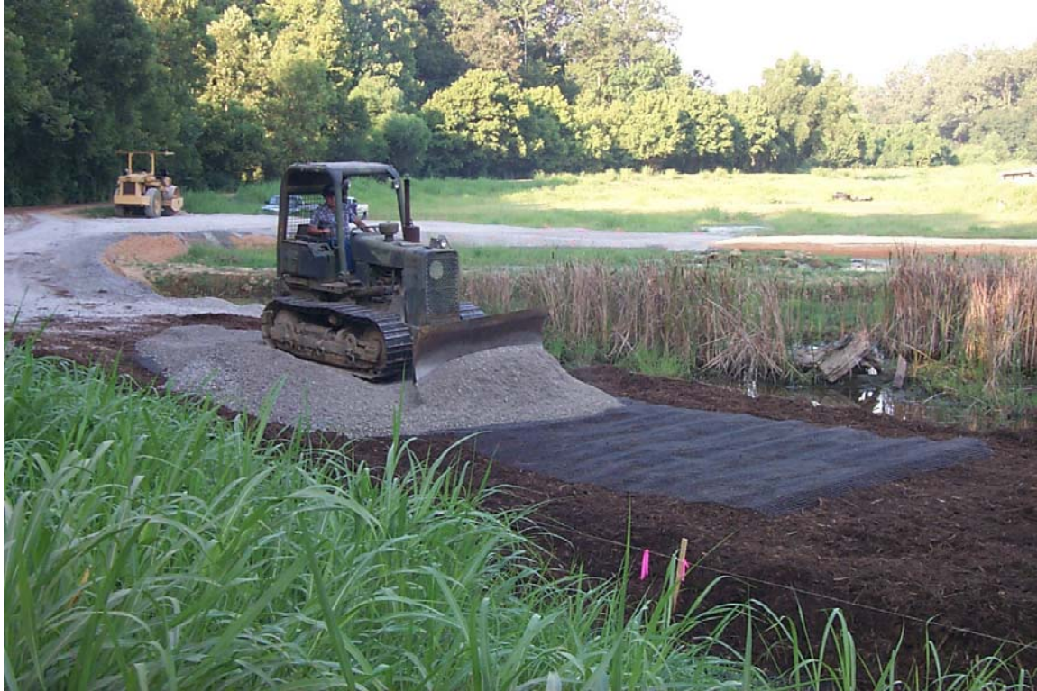
Figure 5. Construction of Item T-2 of soft subgrade test section Santoni et al. 2001 (5)
