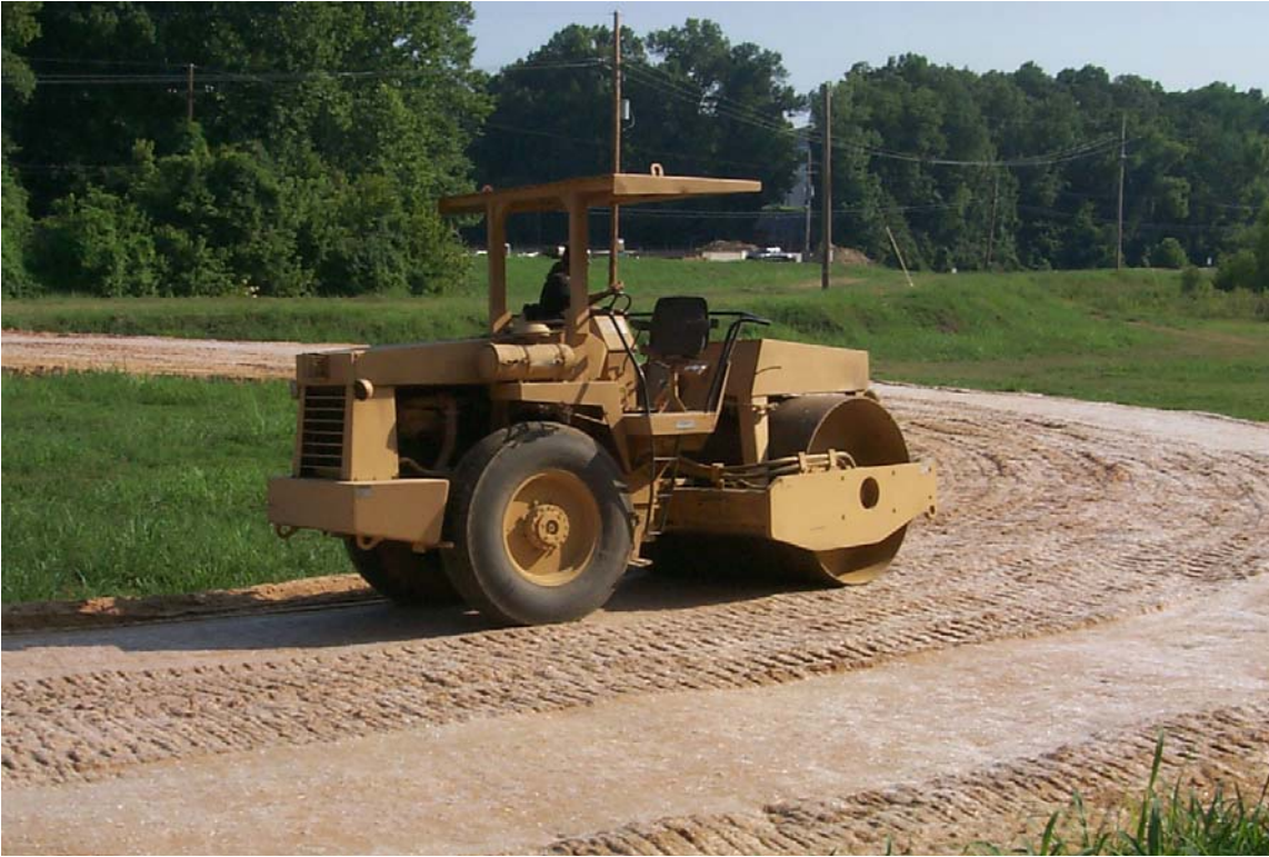
Figure 1. Compaction of geofiber-stabilized sand
