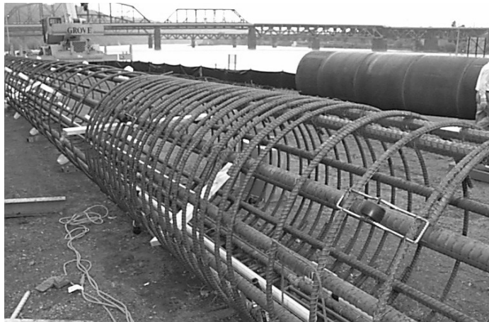
Figure 42. Reinforcing cage for the drilled shaft load test prior to project construction at Braddock Locks and Dam 2
