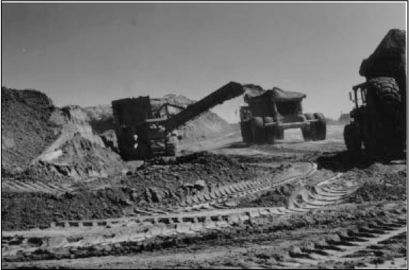
Figure 3-24.—A Holland loader excavating a vertical face mixing silt and fine sand deposits for impervious fill at Reclamation's Calamus Dam, Nebraska (Sept. 1983).
