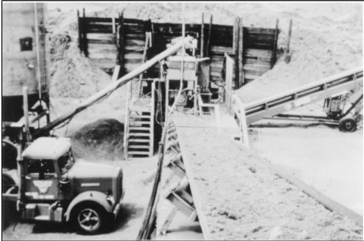
Figure 3-48.—Cement vane feeder and soil feed belt to pugmill at Cheney Dam in Kansas.
