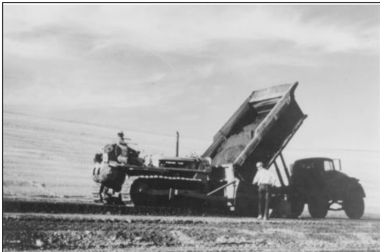
Figure 3-45.—Soil-cement placement at Merritt Dam in Nebraska.
