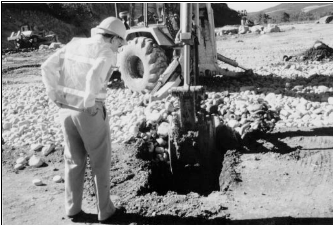
Figure 3-27.—Test pit at the interface of sand filter and gravel drain, Jordanelle Dam, Utah (September 1990).
