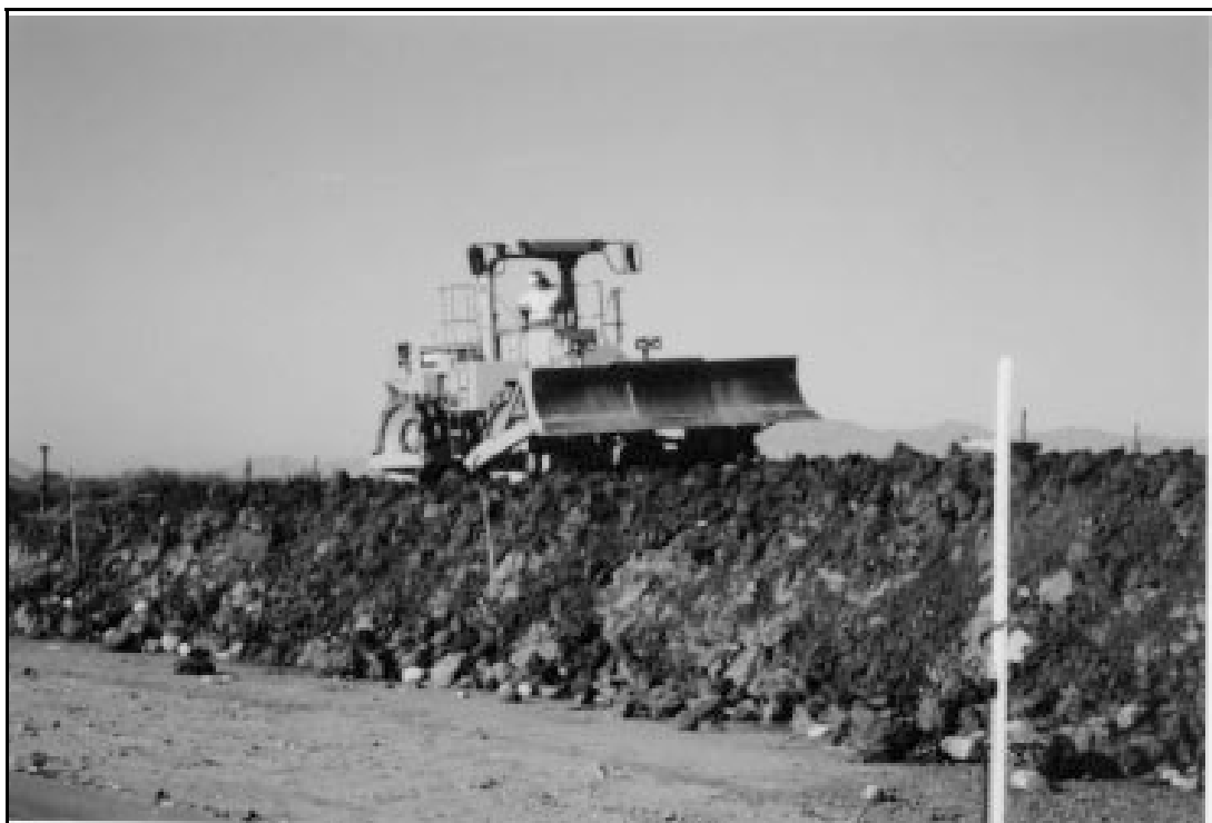
Figure 3-22.—Pad foot roller on a test fill of zone 1 material at New Waddell Dam, Arizona (1990).
