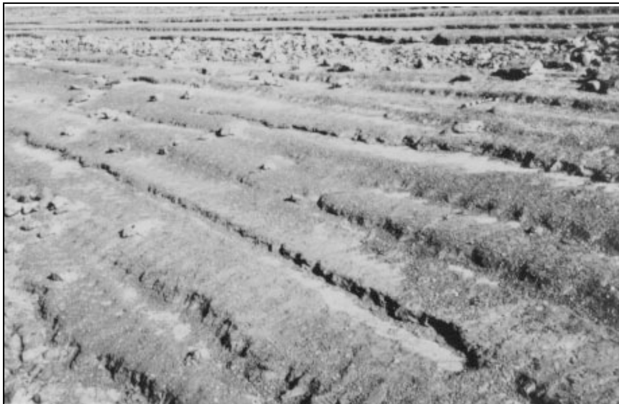
Figure 3-42. — Soil-cement facing at Lubbock Regulating Reservoir in Texas.
