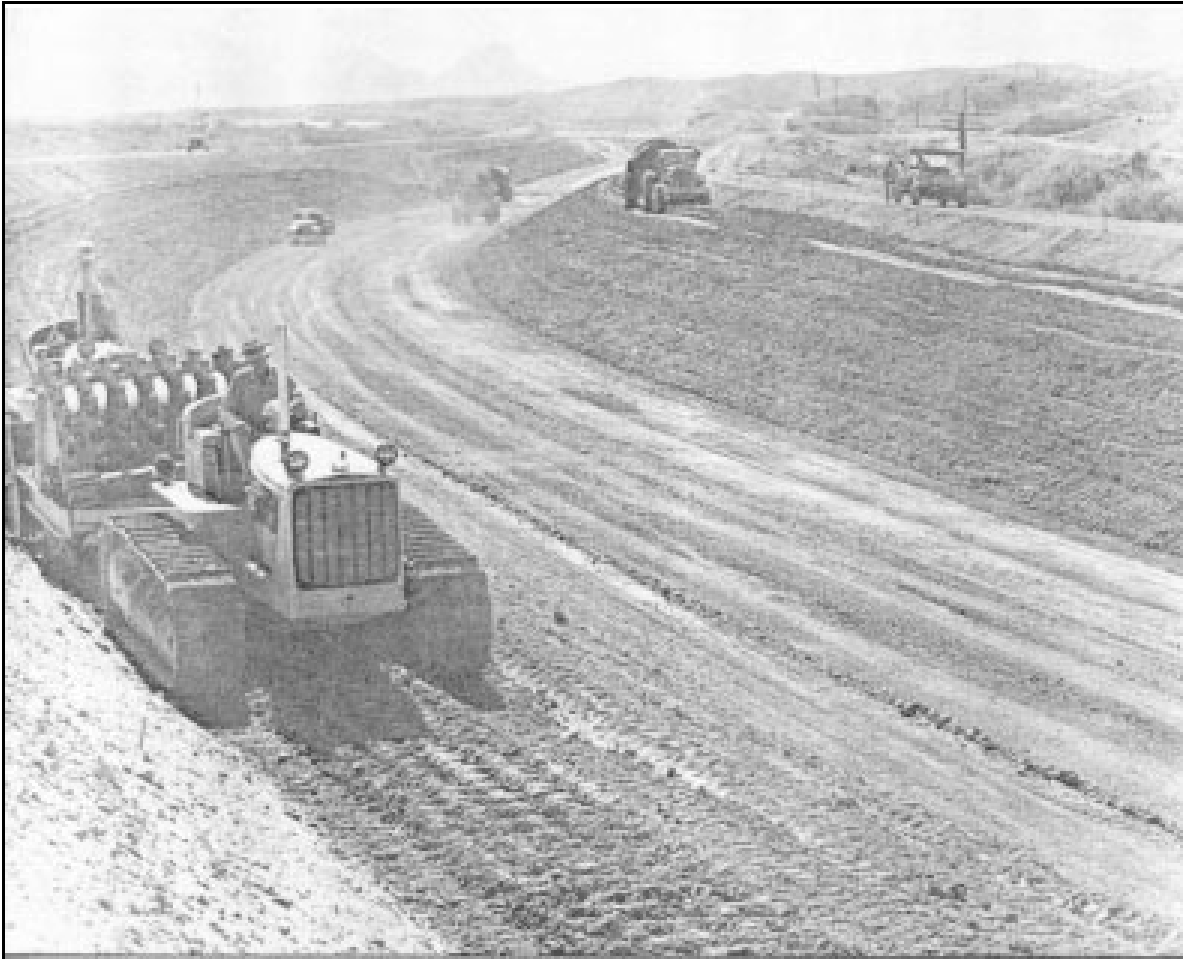
Figure 3-33.—Placing and compacting thick earth lining in Welton-Mohawk Canal in Arizona.
