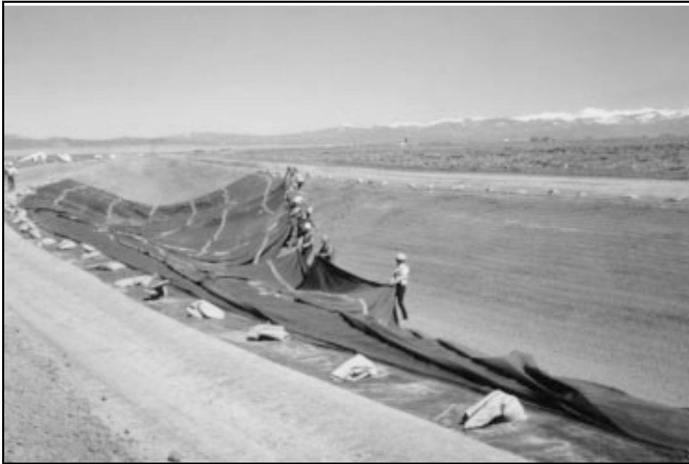
Figure 3-35.—Geomembrane being placed over prepared subgrade.
