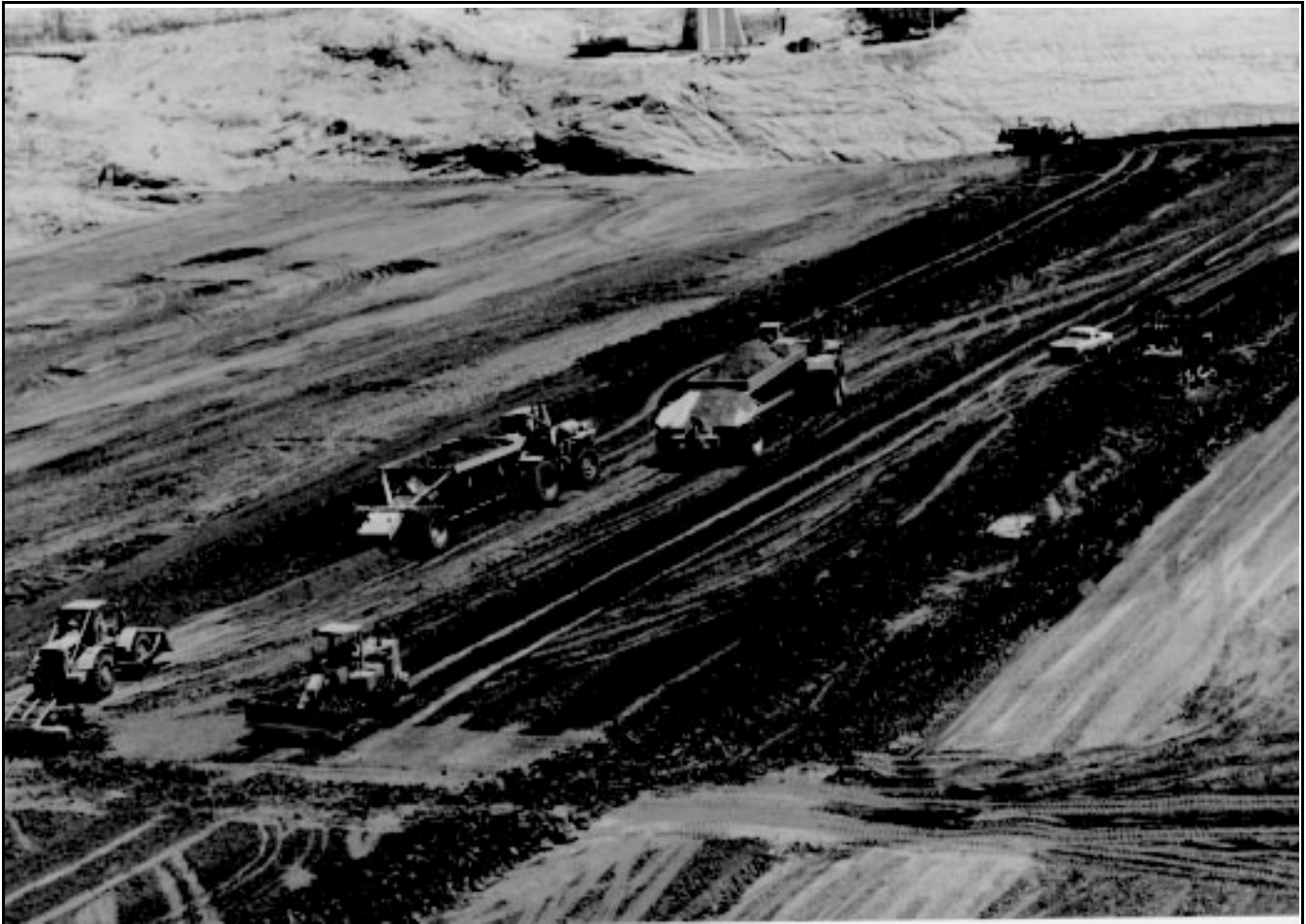
Figure 3-20.—Earthfill operation on impervious zone at Reclamation's McPhee Dam, Colorado. Selfpropelled tamping compactor and disk plow in the foreground. Dart and Caterpillar belly dumps hauling and placing impervious fill in the center of the photo. Contact between filter/drain chimney can be seen on right side (July 1983).
