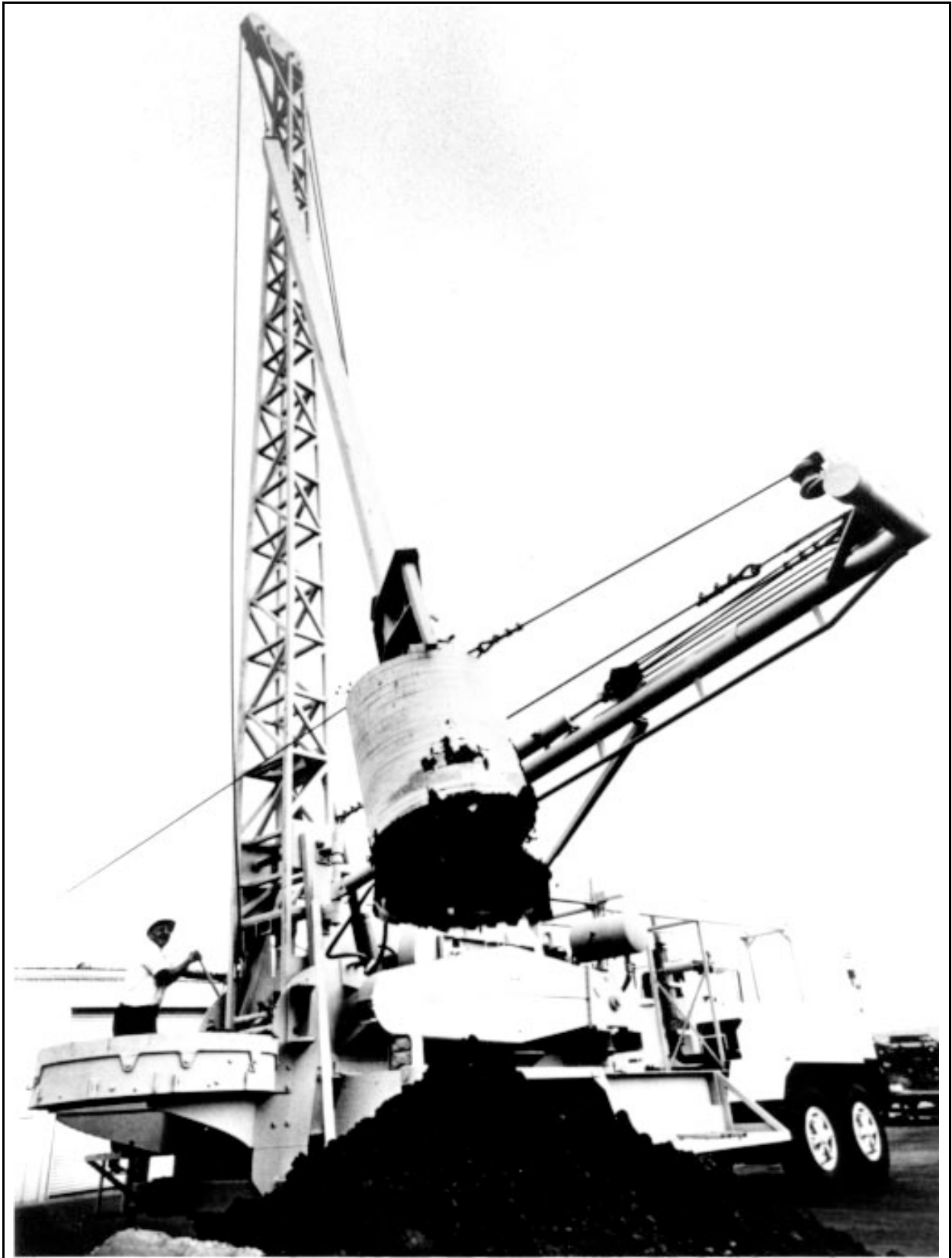
Figure 2-25.—Bucket drill rig in drilling position with a 24-foot triple Kelly and 36-inch bucket.
