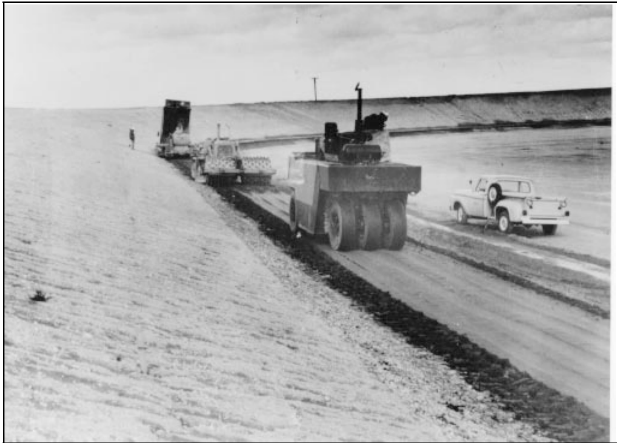
Figure 3-46.—Compaction of soil-cement at Lubbock Regulating Reservoir in Texas.
