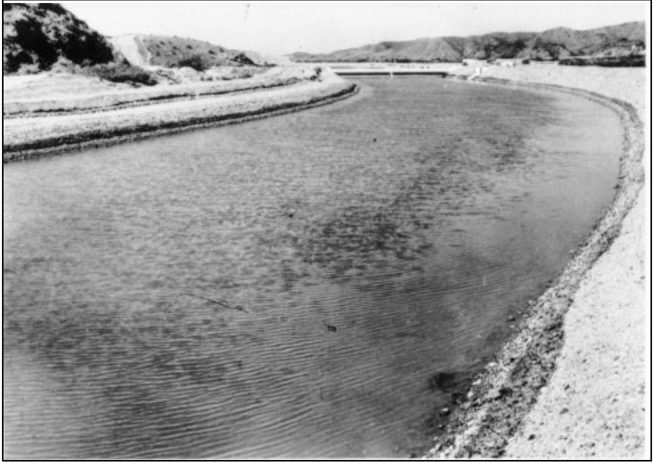
Figure 3-34. — Completed thick earth lining in Welton-Mohawk Canal in Arizona.
