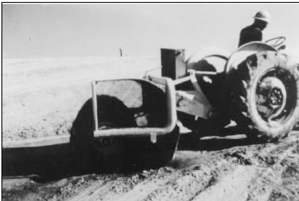
Figure 3-47.—Power brooming of surface prior to placement of next lift at Lubbock Regulating Reservoir in Texas.
