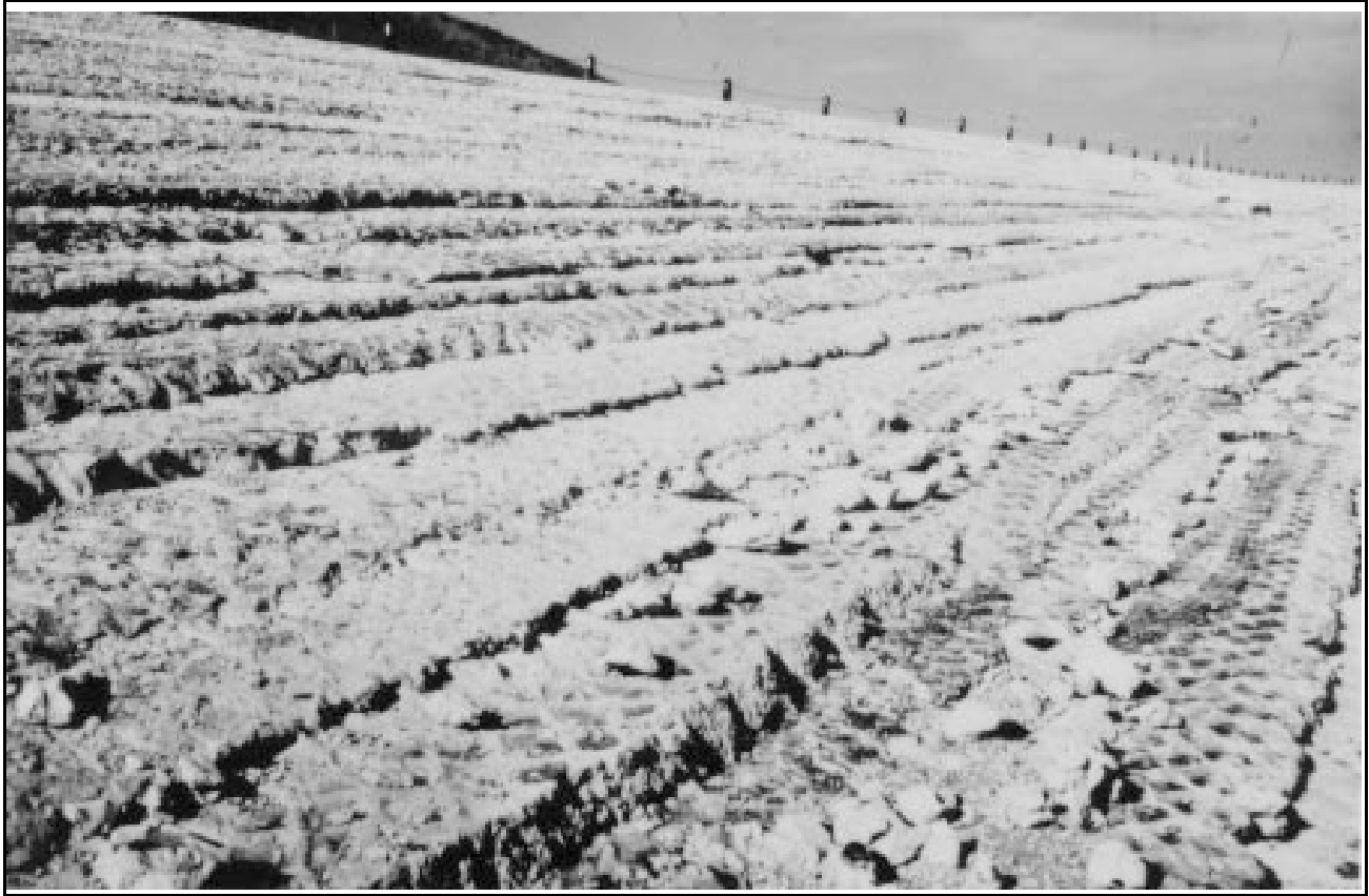
Figure 3-43.— Soil-cement facing at Merritt Dam in Nebraska.
