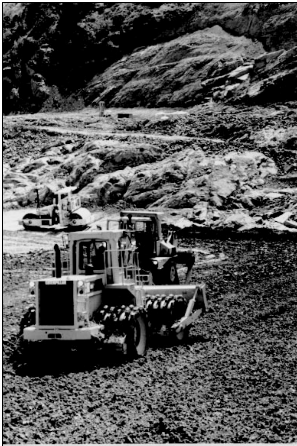
Figure 3-18.—Earthfill (zone 1) compaction by a model 925 C Caterpillar pad foot roller. Also, notice filter upstream of zone 1 being compacted by a vibratory roller. Filter is over weathered fracture zones in the foundation rock (July 1990).
