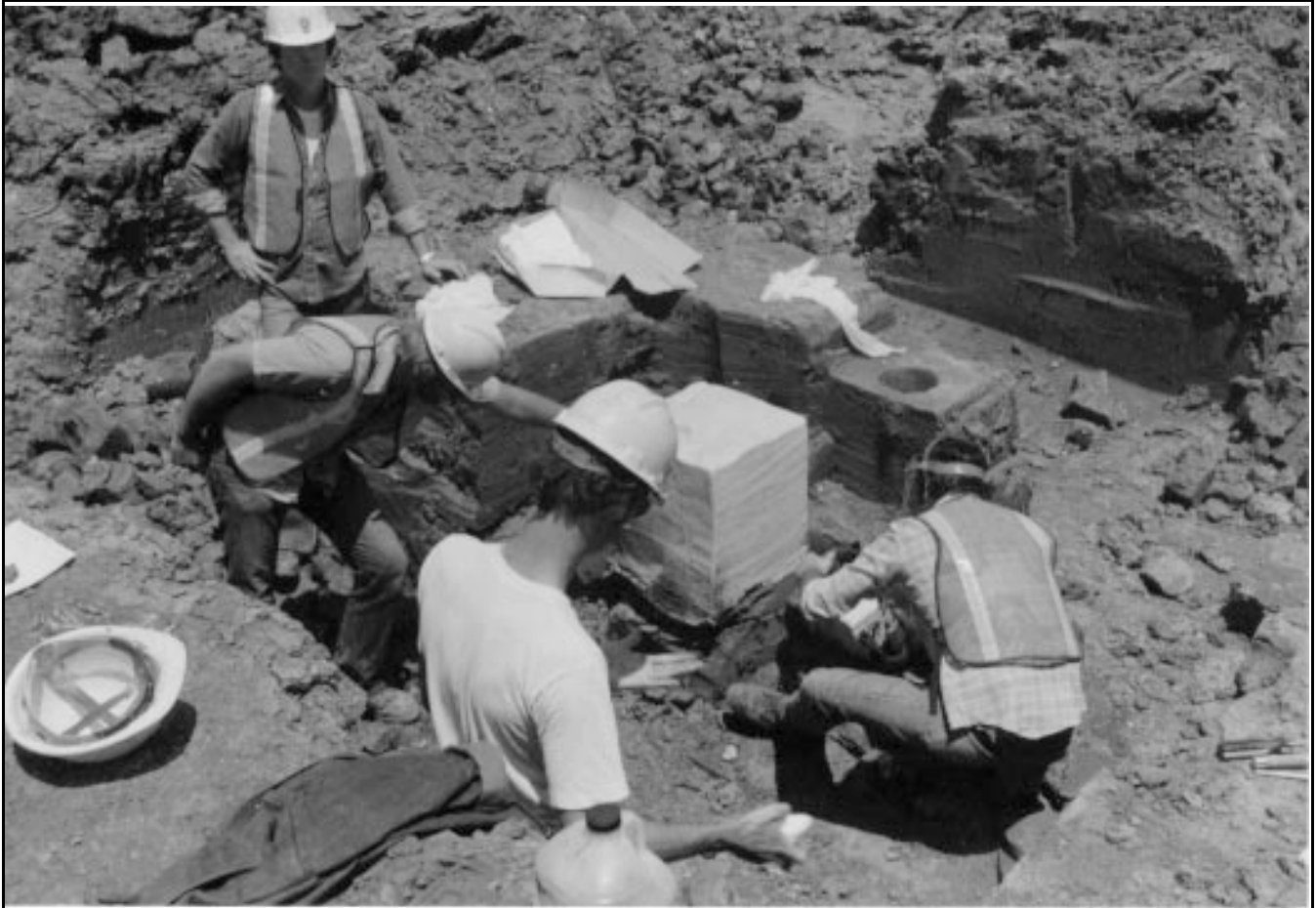
Figure 3-26.—Block sample from test pit in zone 1 at McPhee Dam, Colorado. Final saw cut being made beneath the sample with a chain saw equipped with special tungster carbide bit. Also shows area where an in place density test was taken 600 mm upstream of the block sample (1983).
