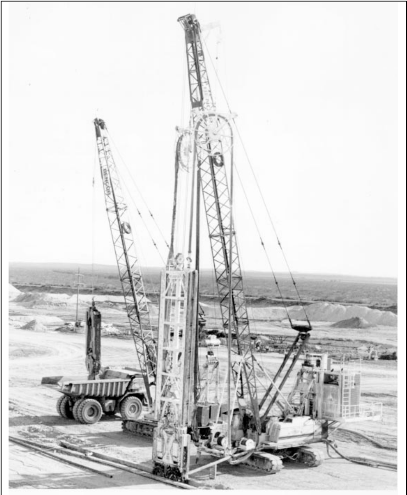
Figure 3-11.—Slurry wall construction using panel excavation and tremie placement—view of a hydromill and crane with 75-cm (30-inch) x 3-m (10-ft) clamshell—Twin Buttes Dam modification.
