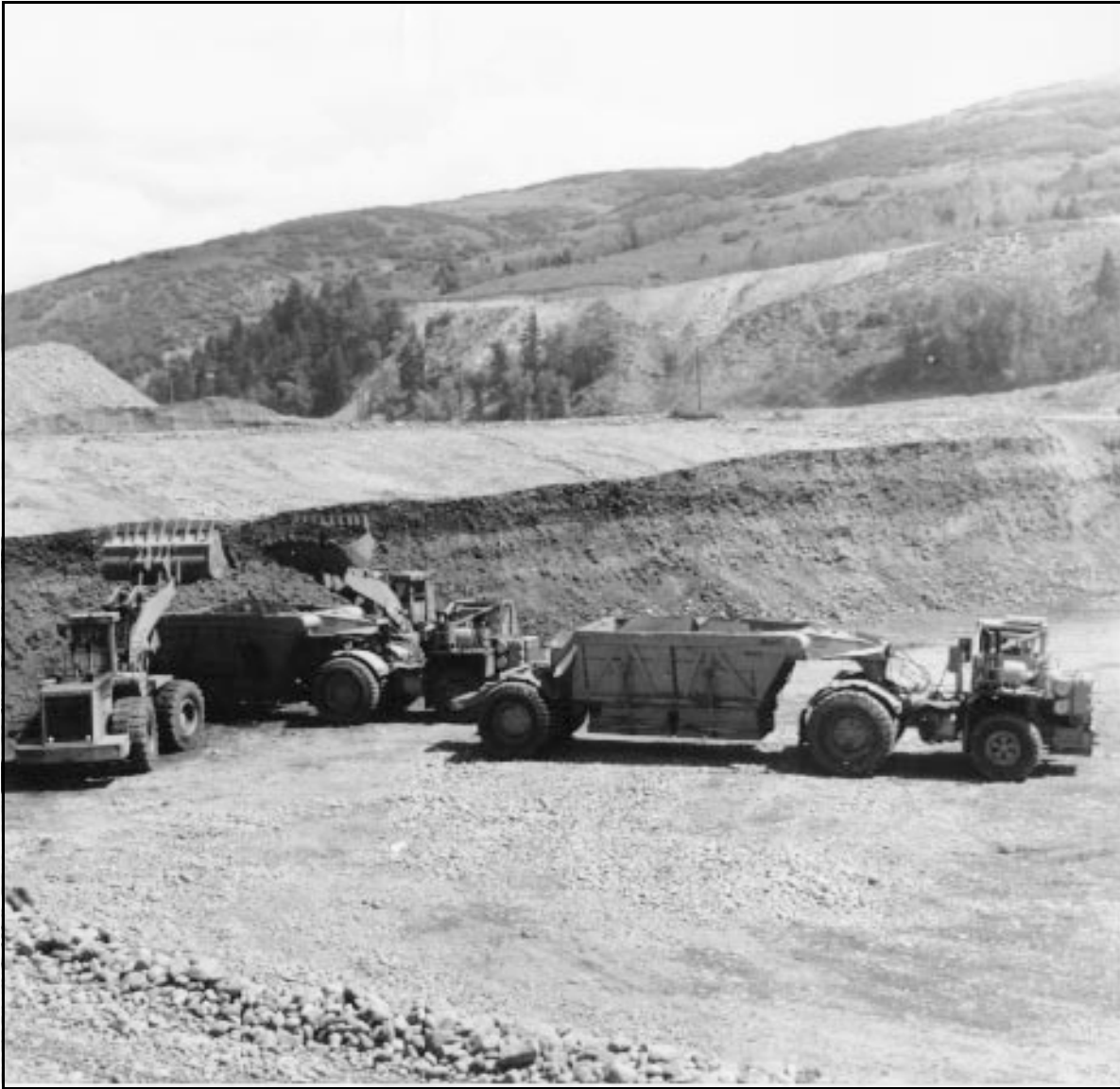
Figure 3-25.—Two model 992C Caterpillar front end loaders loading zone 4 (gravel and cobble fill) from borrow into a model 540 Dart belly dump truck. This type of loading operation, with steep face of borrow area, can be used to get a well mixed fill from a layered deposit. Jordanelle Dam, Utah (August 1990).
