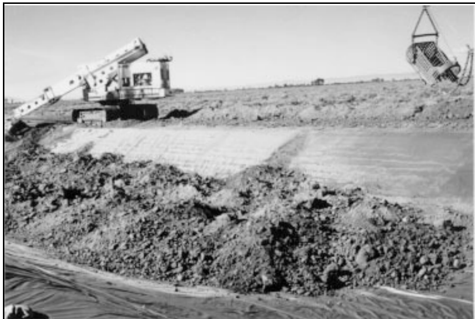
Figure 3-36.—Placement of a protective earth cover over a geomembrane.
