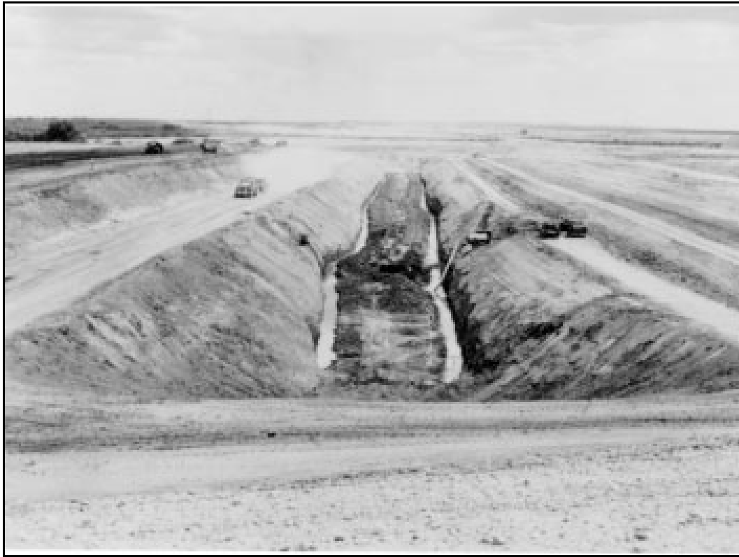
Figure 3-6.—Cutoff trench at Twin Buttes Dam in Texas.
