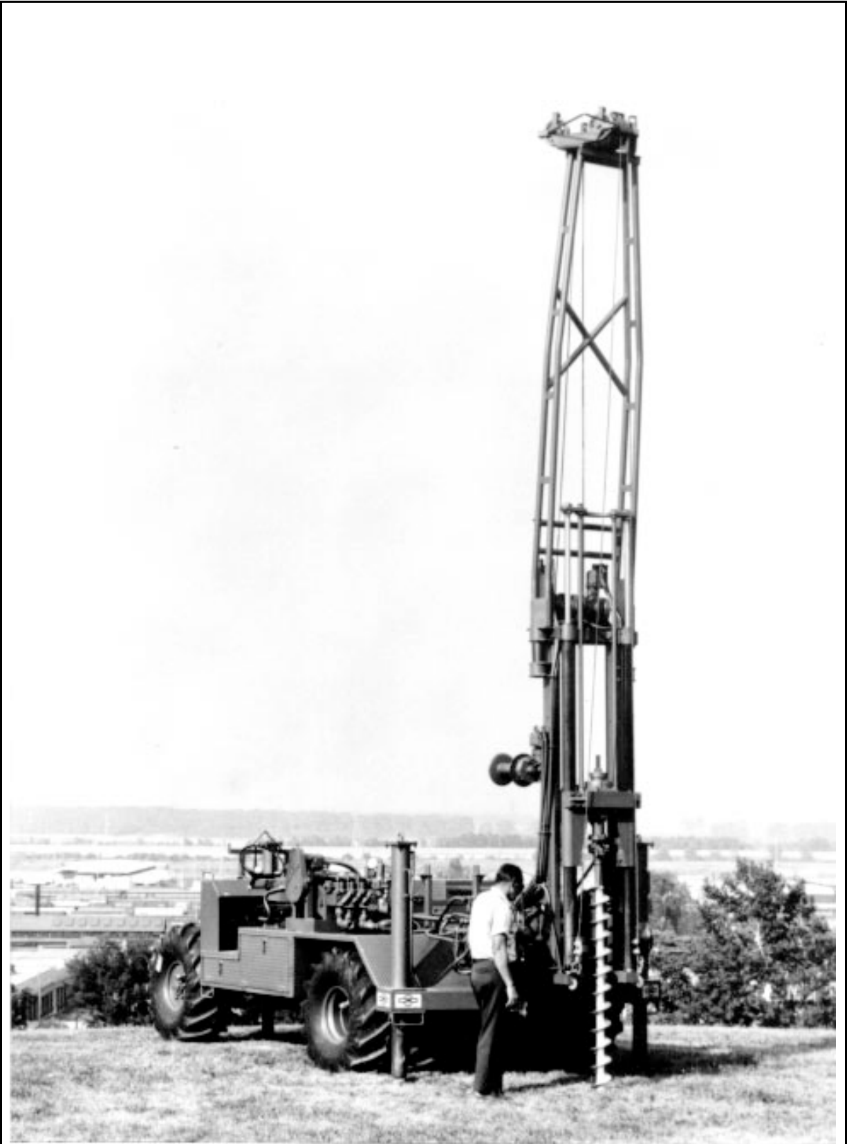
Figure 2-22.—Continuous-flight auger mounted on an all-terrain carrier.
