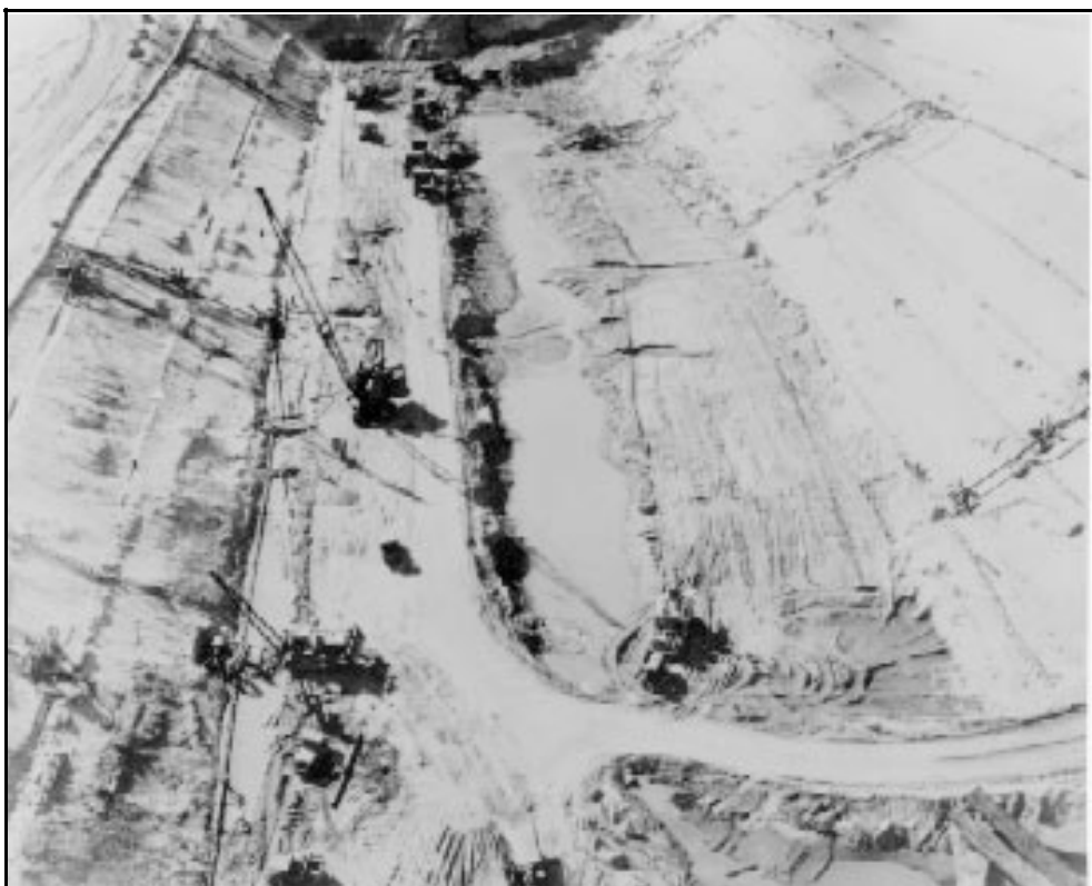
Figure 3-5.—Cutoff trench at Davis Dam in Arizona.
