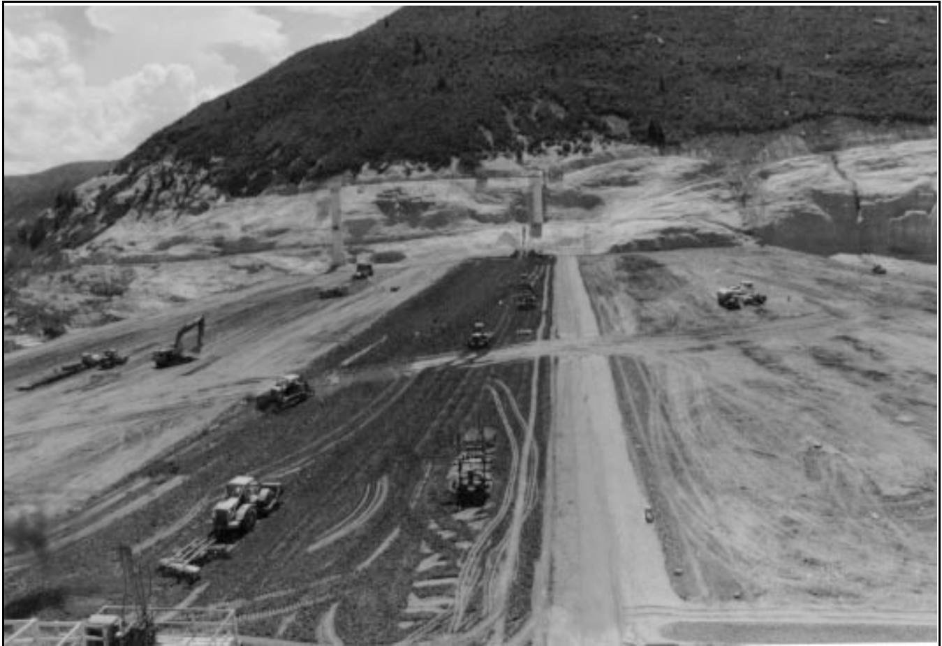
Figure 3-21.—A view of McPhee Dam under construction. Upstream is to the left. Zoning can be clearly seen. From the left: gravel and cobble fill shell; impervious zone 1; zone 2 filter material; zone 2a drainage material; and downstream gravel and cobble fill shell.
