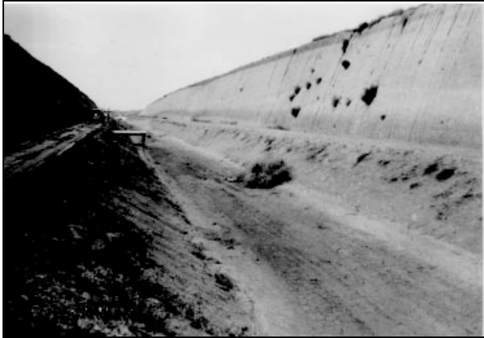
Figure 1-22.—A 34-foot cut on 1/2:1 slope in loess formation— Franklin Canal, Nebraska.
