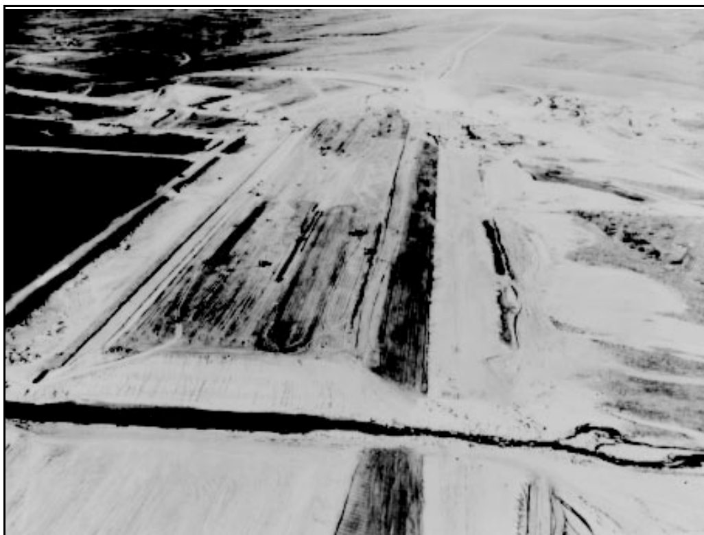
Figure 3-16. —Temporary diversion channel through Bonny Dam, Colorado.
