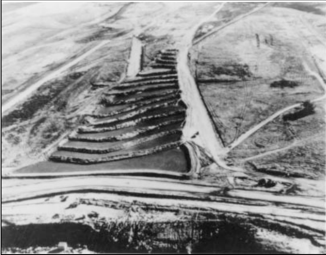
Figure 3-9.—Ponding dry foundation of Trenton Dam in Nebraska.
