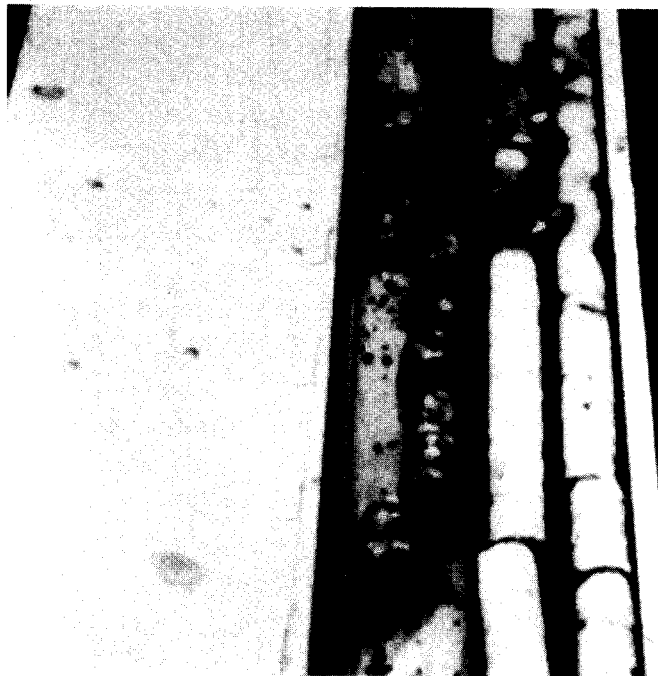
(b) Shaft with defect caused when concrete began to set while removing the casing
