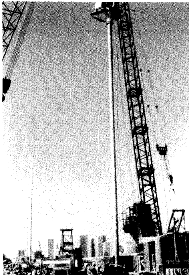
Figure 8.11. Photograph of gravity-fed tremie partially extracted
