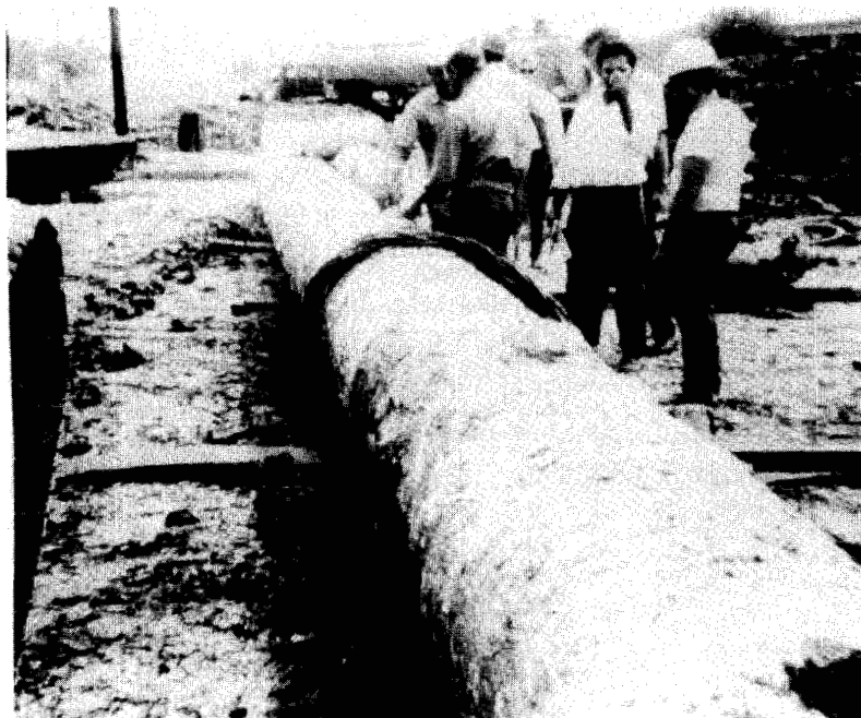
Figure 8.19 b. Drilled shaft of excellent quality after exhumation
