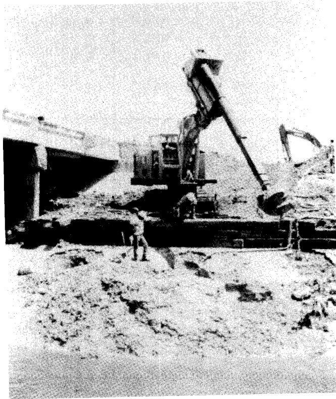
Figure 4.4. Low-headroom drilling machine (crawler-mounted) (Photograph courtesy of A. H. Beck Foundation Company)
