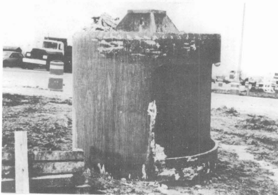
Figure 4.6. A typical "muck bucket" or "clean-out bucket"
