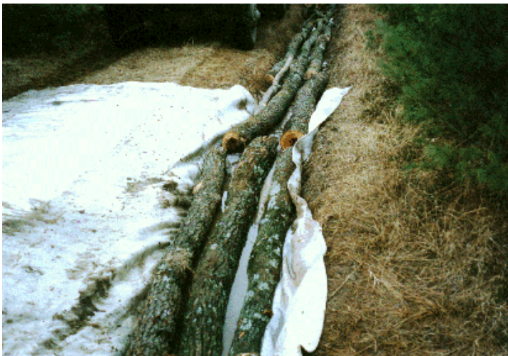
b. Larger diameter logs used to fill large rut.
