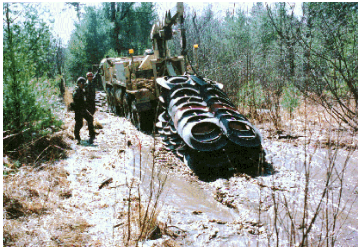
Figure 5. Placing tire mats onto wooded trail section.
