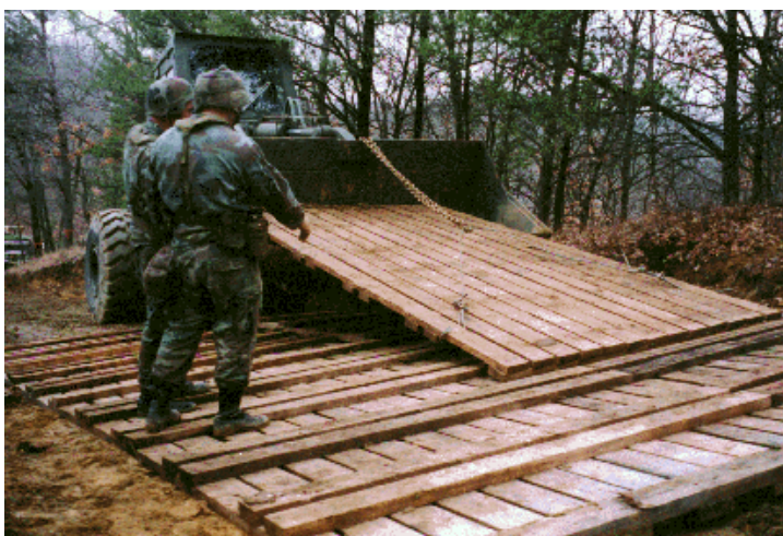
Figure 3. Lifting Uni-Mats with bucket loader.
