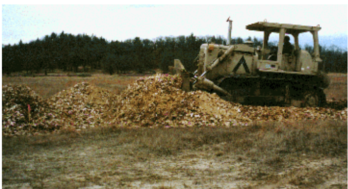
Figure 7. Spreading fill material with D7 bulldozer.
