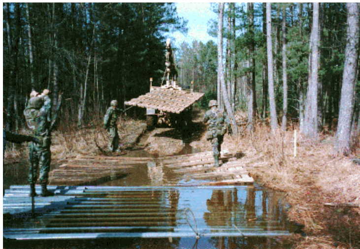
Figure 4. Placing Uni-Mats in wet site.
