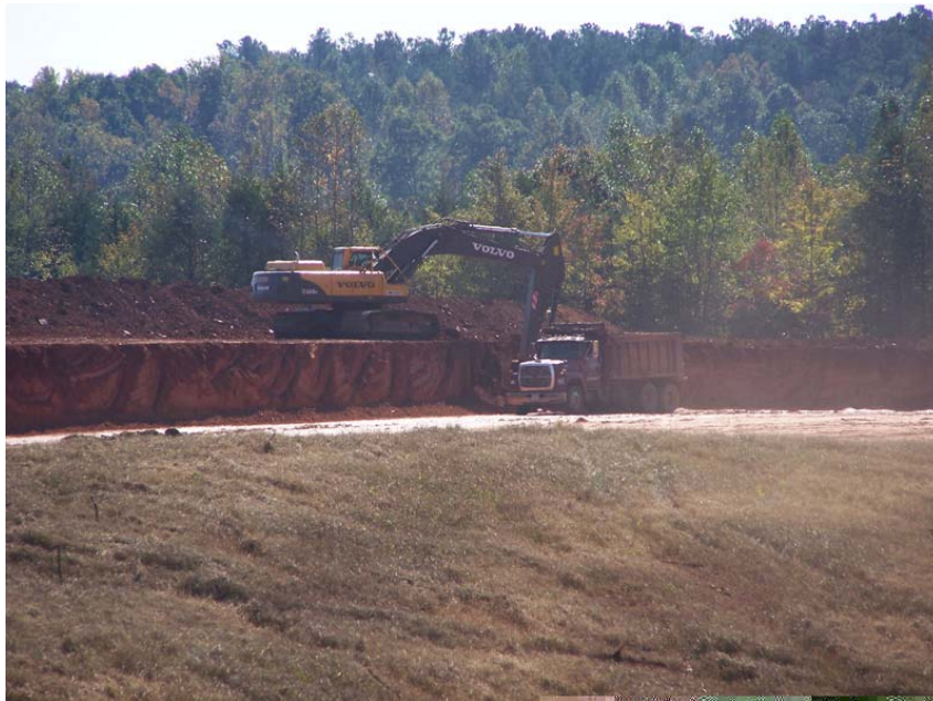
Figure 6.4 - Vertical excavation of soil onsite
