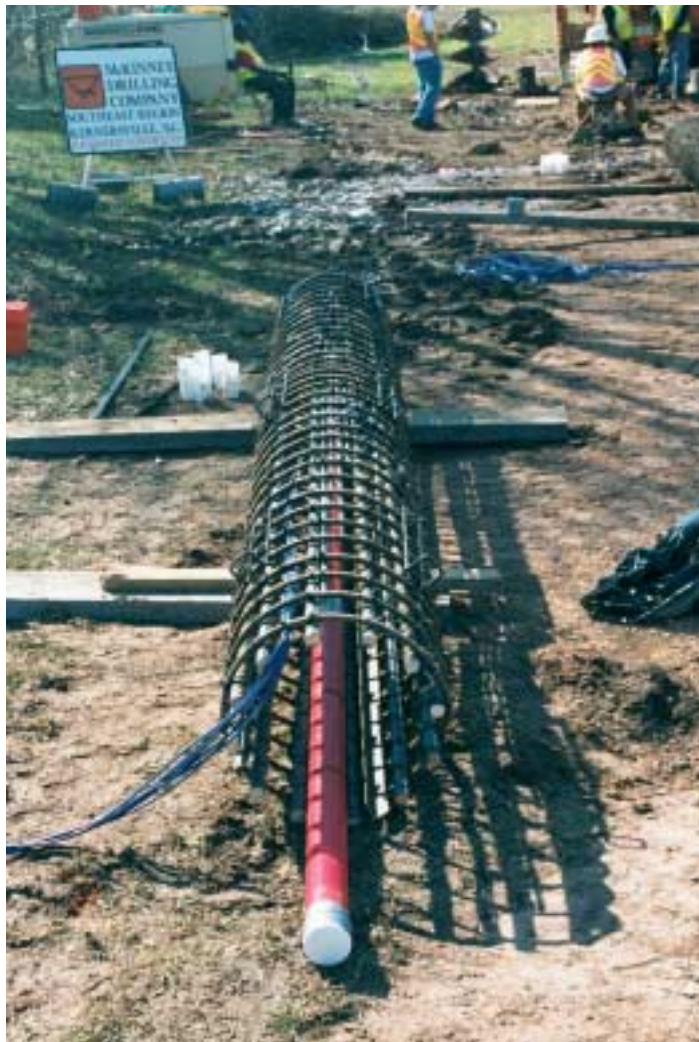
Figure 100. Instrumented Reinforcement Cage
