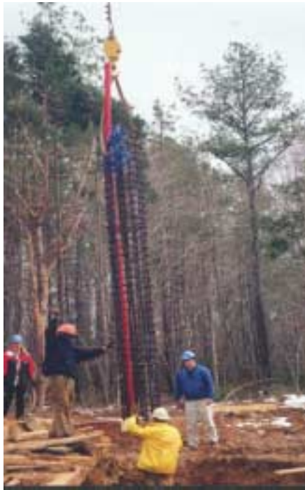
Figure 33. Installation of Steel Cage
