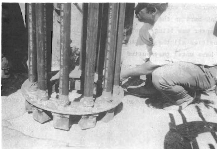
Fig 6.12. Plastic tube pushed into the steel stub and cloth tape wrapped around it.
