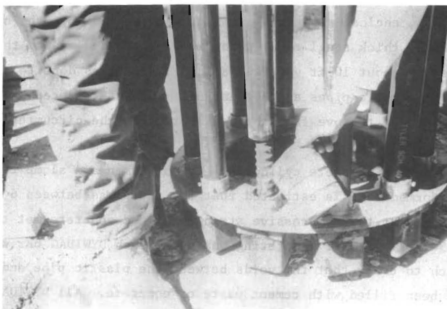
Fig 6.11. Molten wax being poured into the steel stub around the DYWIDAG bars.
