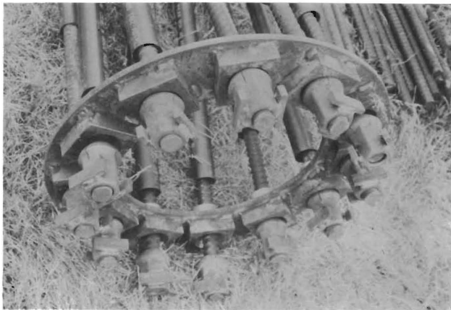
Fig 6.9. DYWIDAG nuts with "ears" at bottom ends of DYWIDAG bars.
