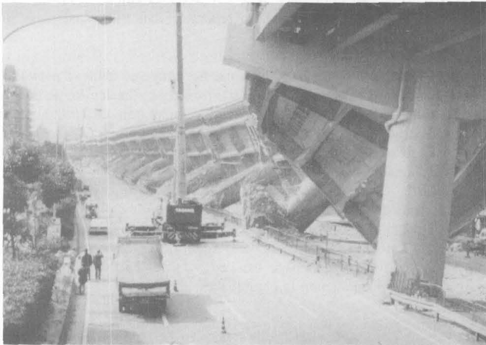
Figure 5. Collapse of Hanshin expressway during the 1995 Kobe (Hyogo-Ken Nabe, Japan) earthquake.
